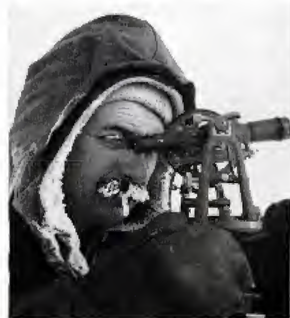
SHOOTING THE SUN Albert Cary fixes the position of the floating ice island. The stars are invisible during the continuous northern daylight.
